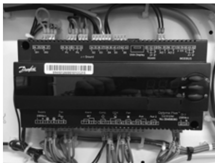
Picture 3 : Normal wiring
